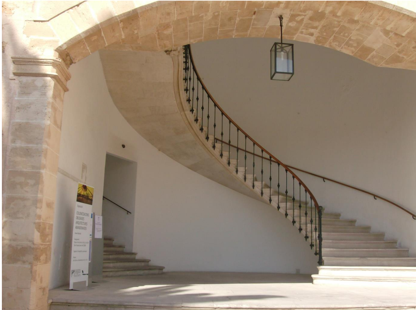
elliptic “cantilever” stone staircase, Palma, 19 th century
