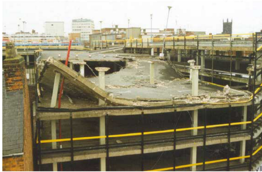
Figure 22: Collapse of Pipers Row car park – mainly a shear mode of collapse. [12]
